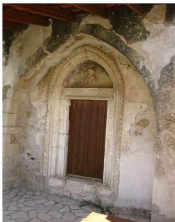
IMG_5559 Panagia at Monochoro near Galia: west door with ruined narthex in foreground
