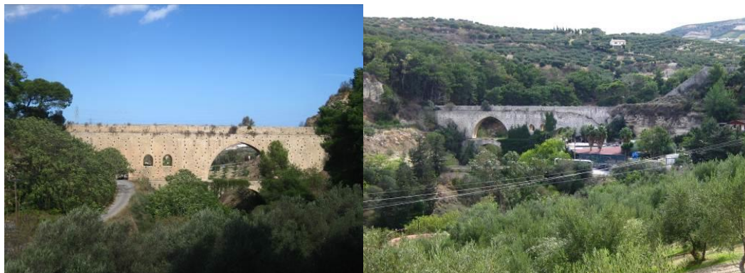
(left) IMG_2731 The aqueduct (Dawkins' no. 1) that was built (or restored) under Egyptian rule in 1839. 29
