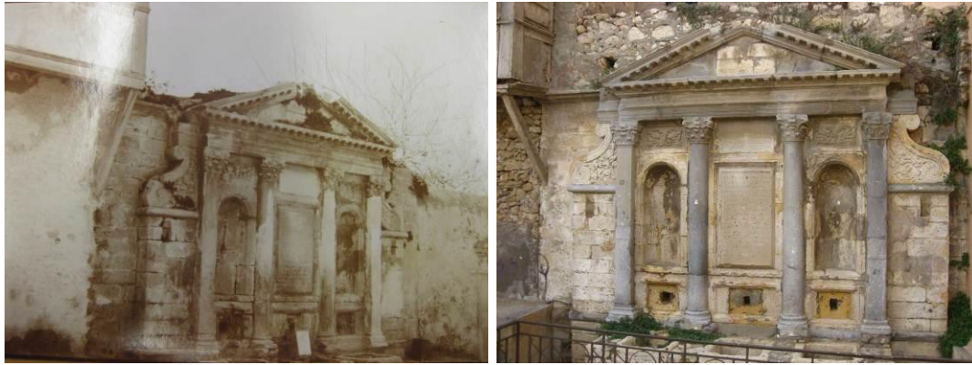
(left) Priuli fountain (photo in Dawkins archive) (right) IMG_2742 (19 Oct. 2010). The wooden beam supporting the overhanging first-floor balcony of the next-door house was still there – just – in May 2011
