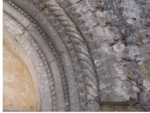
IMG_8078 Moulding on W door
