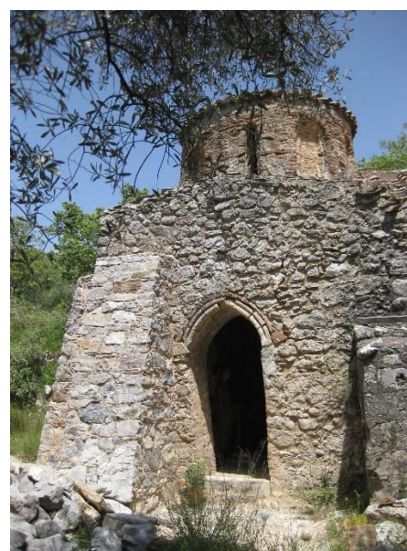
IMG 0342 (21/4/09) St John below Gerakari, now re-roofed and somewhat restored
